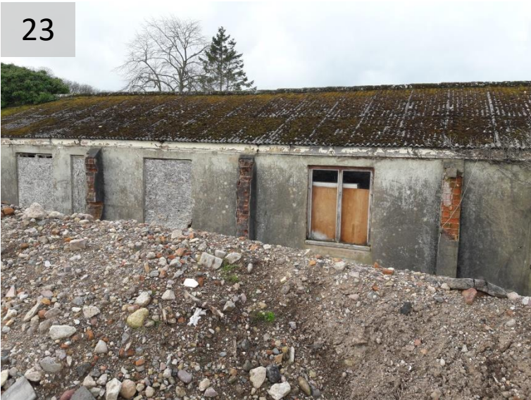
Asbestos cement corrugate roofing.
