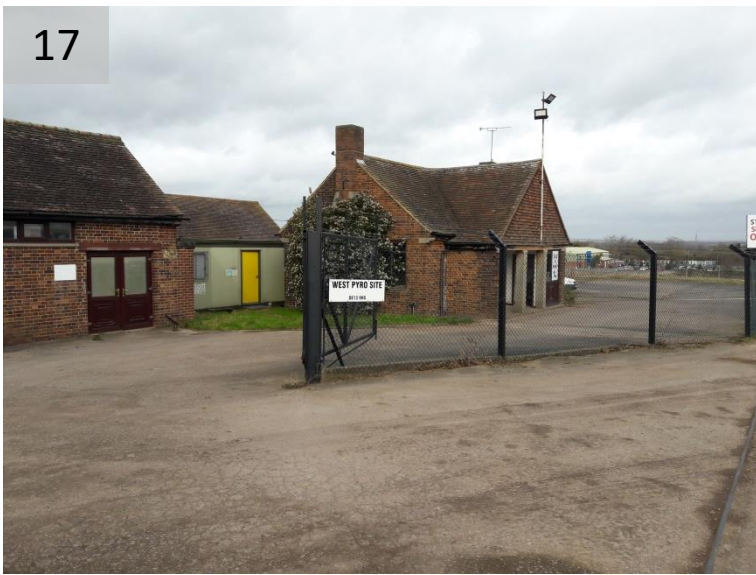
Site offices and firework storage buildings. View west.
